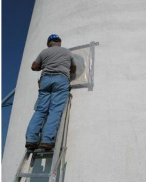
Sealing opening (photo: Oklahoma State University)
