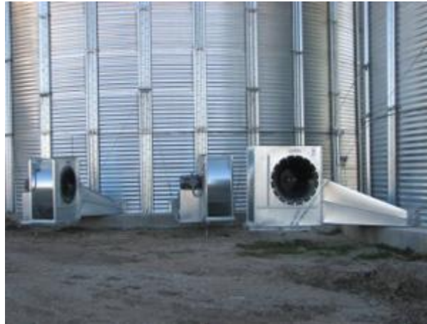
Bin aeration fan (photo: Feed&Grain.com)
