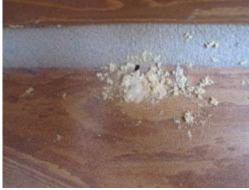
Fresh powderpost beetle activity (image: volvoab.com)
