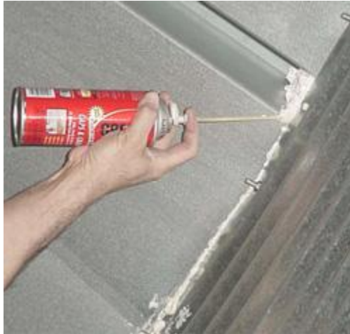
Sealing seams with silicone caulk (photo: factsheets.okstate.edu)
